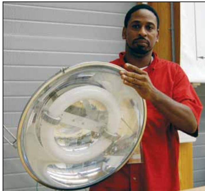
Engineering technician Alfie Brown holds one of the lab's new induction lights, installed high over the Ion Cyclotron Resonance lab. Because the lights themselves have tiny magnetic fields of their own, they can only be used in labs with very high ceilings. Photo by Amy Mast
